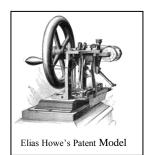
*Scientific American* promptly published the patent claims on September 26, 1846, under the heading "New Inventions."<sup>68</sup> Howe's three elements formed the core of the Singer Sewing Machine that would eventually sweep the United States in the 1850s.
